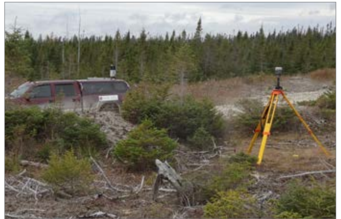
Before setting out, the team first set a control point and collected two hours of data with a Trimble R10 GNSS receiver.
